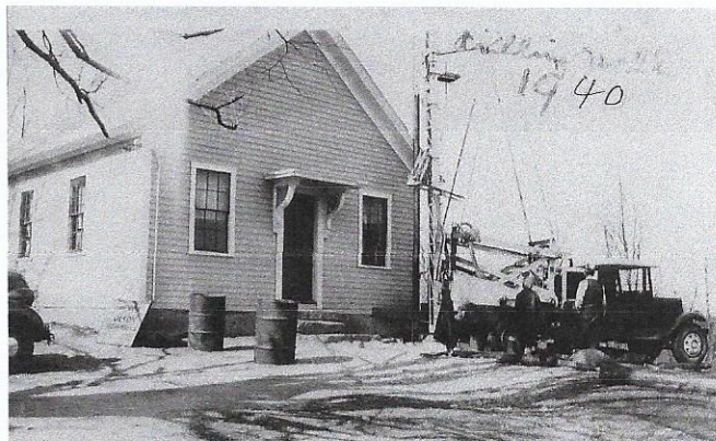
New Well Being Drilled in 1940
