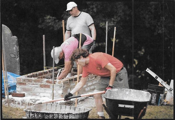
Rebuilding the crypt
