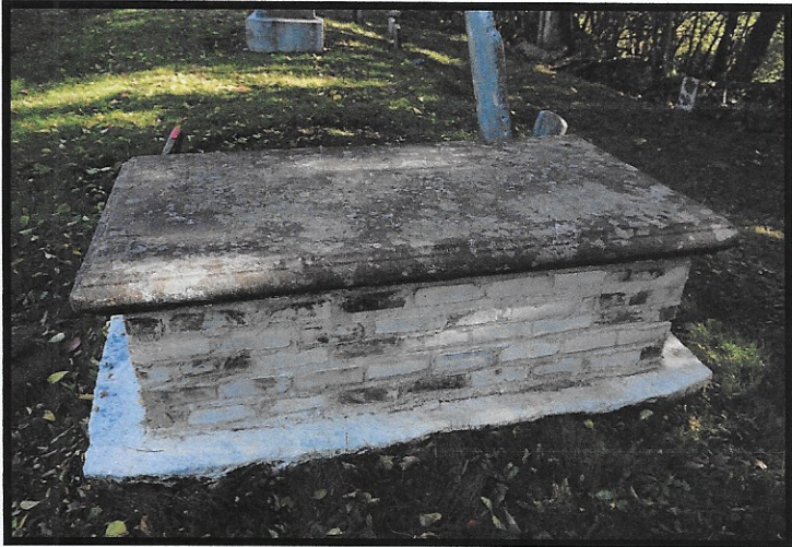
The finished restored crypt
