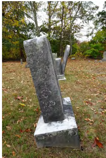
1. Artemas Fuller monument is leaning and ready to slide off the base.
