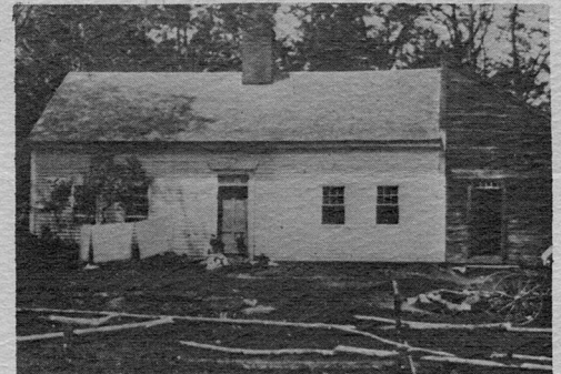
John C. Dudley house on Buttonwood Avenue before renovation in 1920
