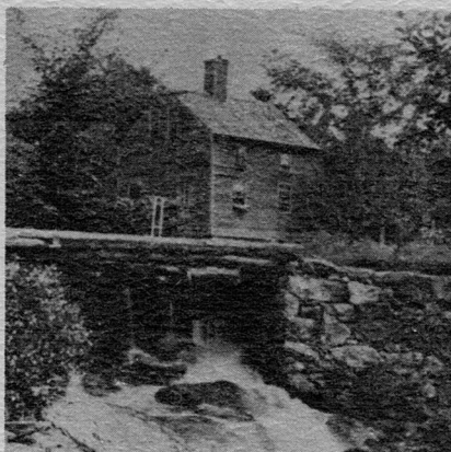
Spillway of Houghton Grist Mill Pond. House moved to Blackstone in early 1900's
