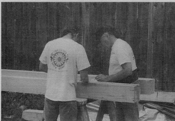
Greg Wolodkin (left) and Steve Colonies measure out a piece of the frame.
