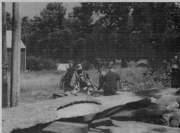
Work carries on at the site.
