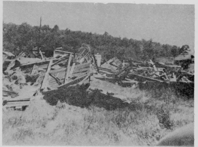
John D. Brigham barn demolished
