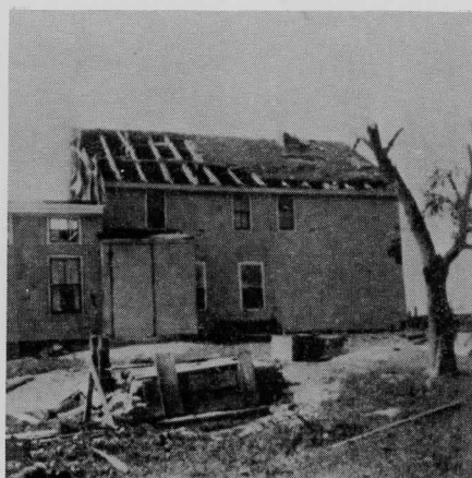
Kratschman Farm main house roof
