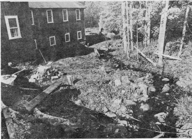
Down Stream from Dam with corner of house and shop to left.
