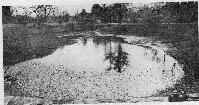
Pond from Dam
