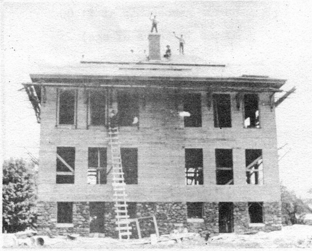
BUILDING THE OLD HIGH SCHOOL
